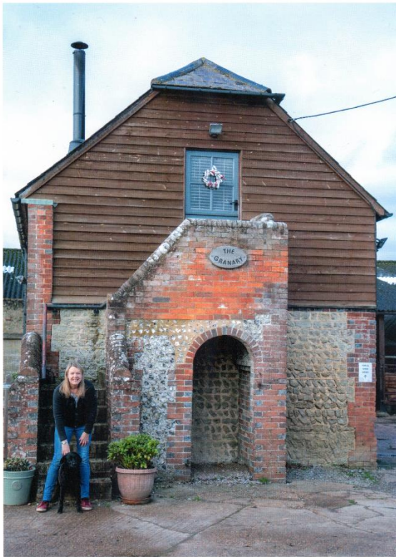
The Granary at Mill Farm
